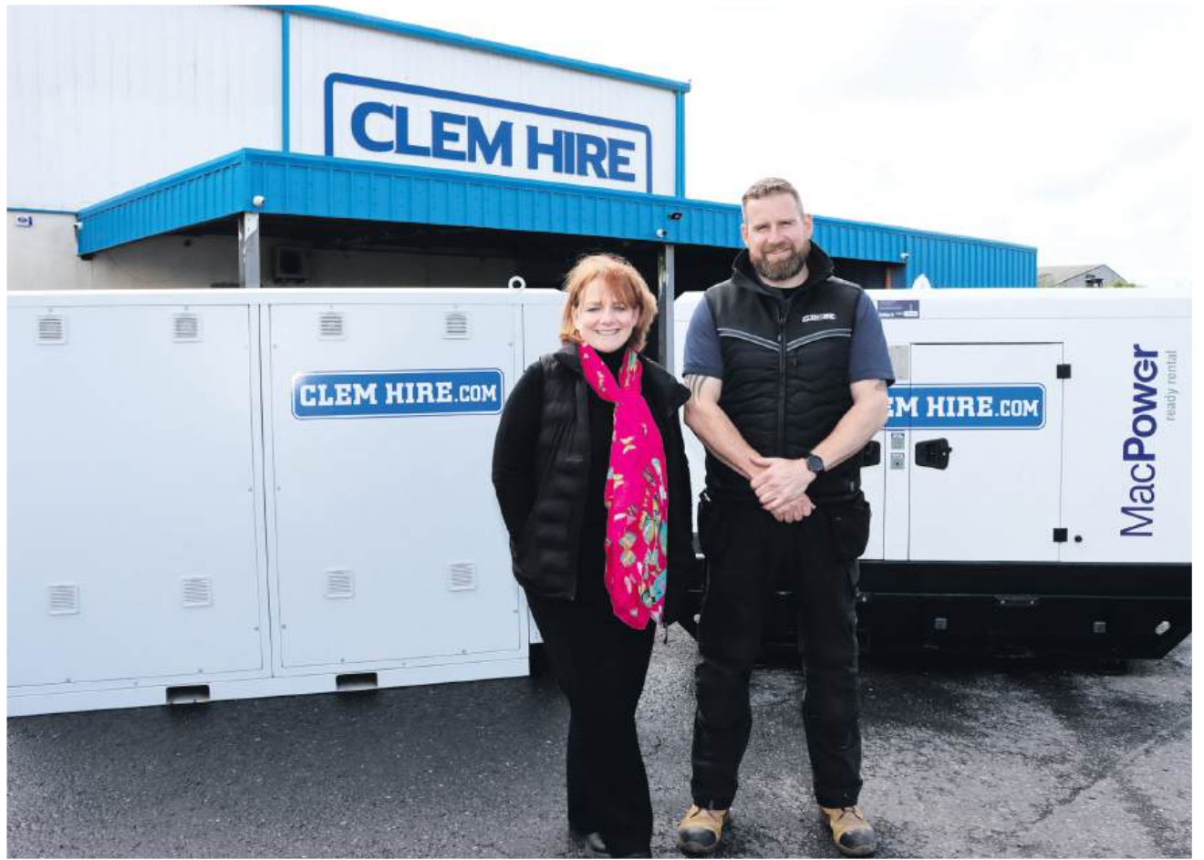
Carmel Jacob, Training Co-ordinator, Clem Jacob Hire, with Pat Walsh, Operations Manager at Clem Jacob Hire, pictured with a battery energy storage system (left) and a standard HVO (Hydrotreated Vegetable Oil) run generator (right).
